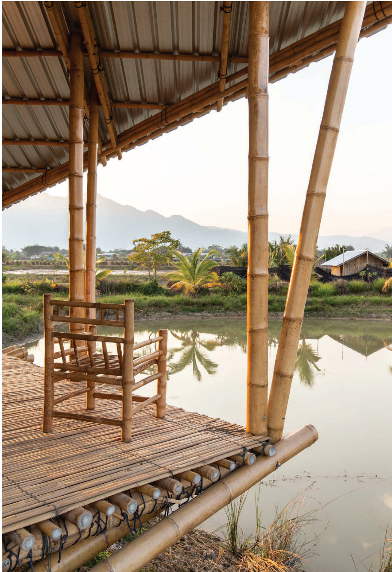
Bamboo is a locally available CO 2 storage resource for construction. The guest house is designed and built by BASEhabitat students, Thailand (2022). Credits: Paul Eis
