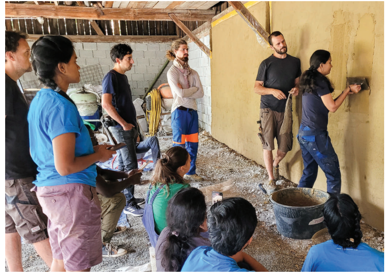
Materials science in theory and practical application during a clay plastering workshop with site manager Dominik Abbrederis in Zöbing, Austria (2022). Credits: Marta Rota
