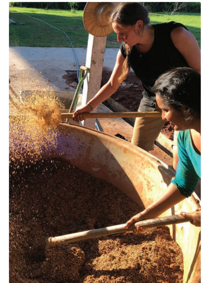
Hands-on experience in Baan Doi, Thailand: preparation of the adobe mix.
