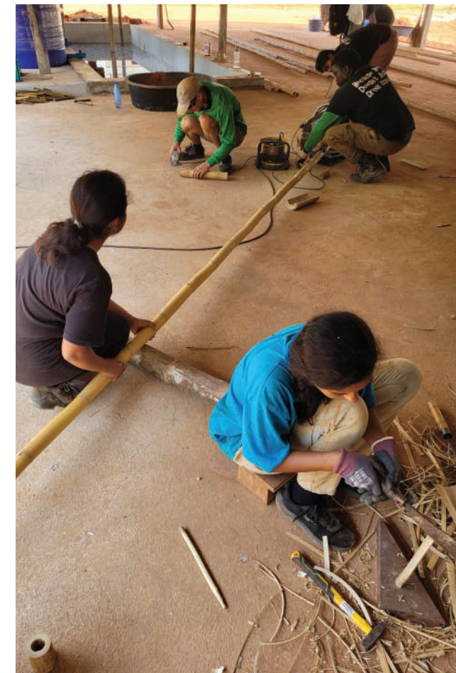
Hands-on experience in Baan Doi, Thailand: bamboo preparation.
